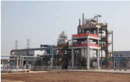
Changmao Lianyungang – Maleic anhydride production line with annual capacity of 10,000 tonnes using butane production method
