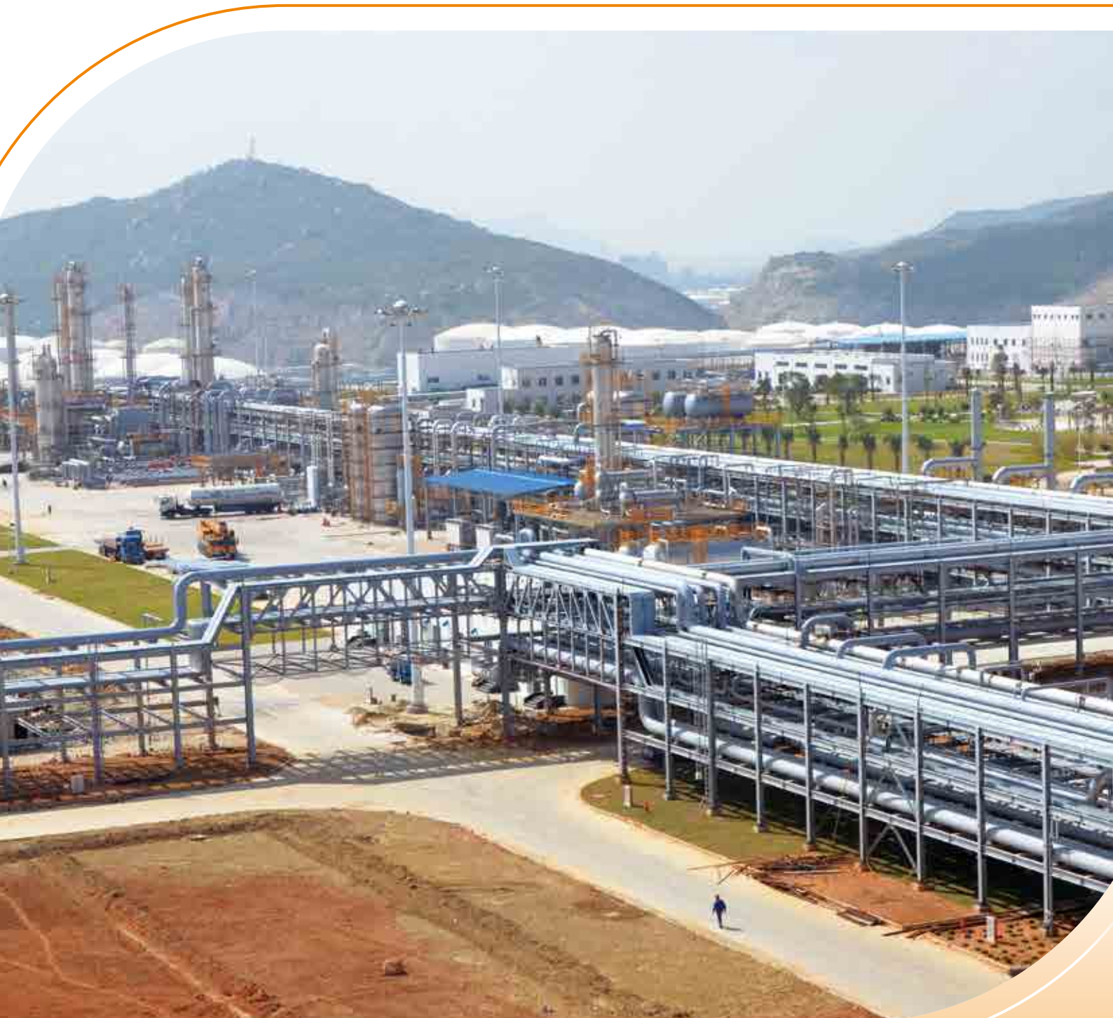
The Gaolan Gas Terminal, in the Mainland, processes the gas and gas-liquids from Liwan 3-1 and Liuhua 34-2 fields.
