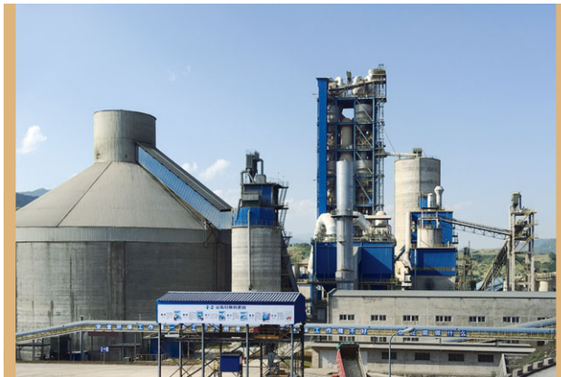
Cement production plant of Puer Kungang & K. Wah Cement Construction Materials Co. Ltd. in Zhenyuan, Yunnan
