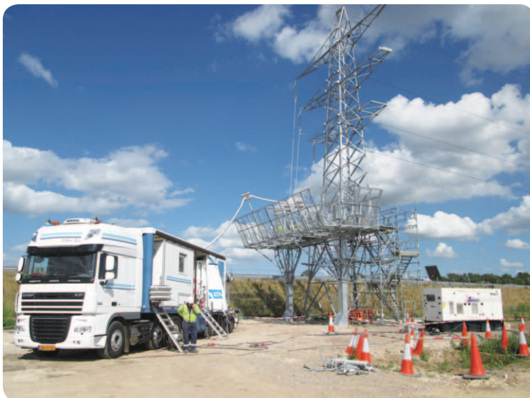
UKPN undertaking works on a Powerline diversion over the M1 motorway.
