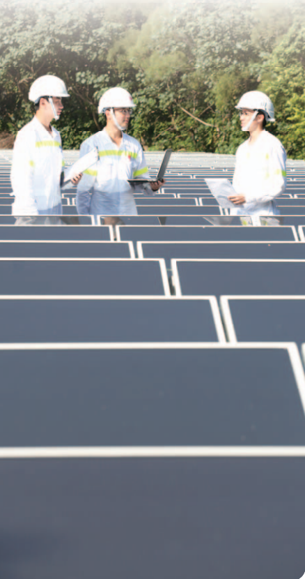
HK Electric's 1-MW solar power system comprising 8,662 thin-film photovoltaic panels is one of the largest in Hong Kong.
