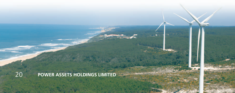
Iberwind's Sra. da Vitória wind farm generates clean energy for Nazaré district.
