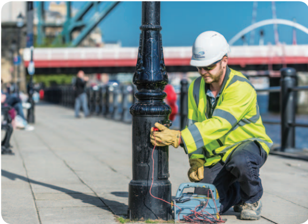
NGN engineer using a wireless sensor to locate underground apparatus.
