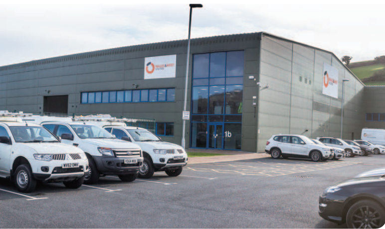
WWU's Colwyn Bay depot upgrades to serve the North Eastern Wales community better.
