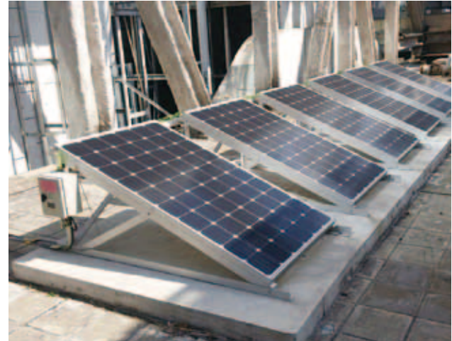
Installation of Solar Panels
