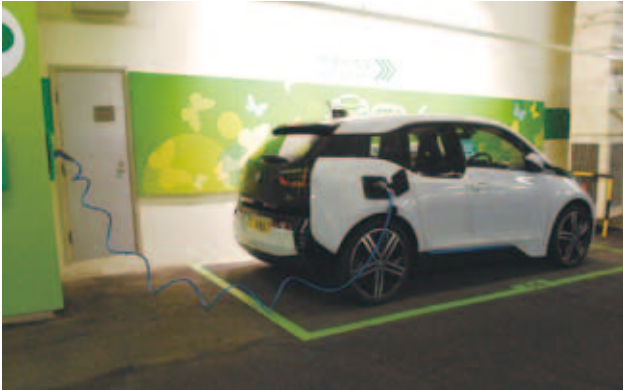
Upgrade of EV Charging Station
