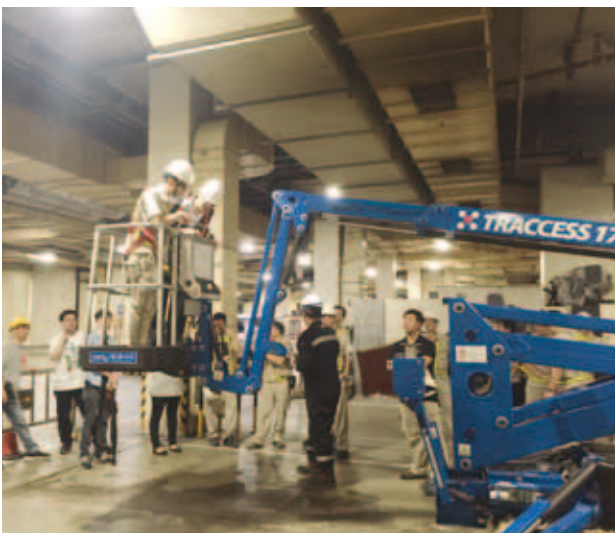
Field Demonstration of Using Aerial Working Platform
