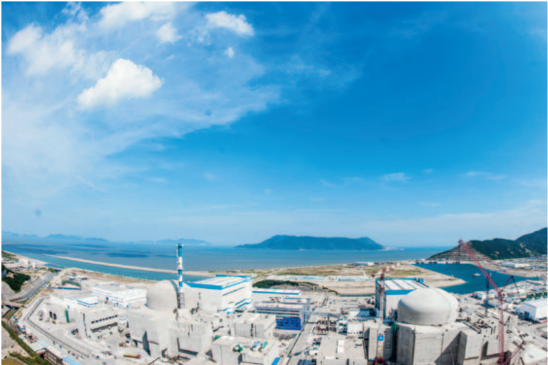
Taishan Nuclear Power project under construction
