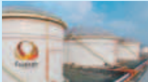
Fujairah Oil Terminal, United Arab Emirates, Middle East 34 storage tanks Storage capacity: 1.155mm m 3
