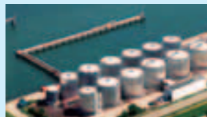
Vesta Terminal Flushing, Holland, Europe 27 storage tanks Storage capacity: 388,500 m 3
