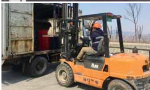
Collection of phosphate waste by a contractor licensed by provincial environment protection bureau at a factory in Ningbo, China
