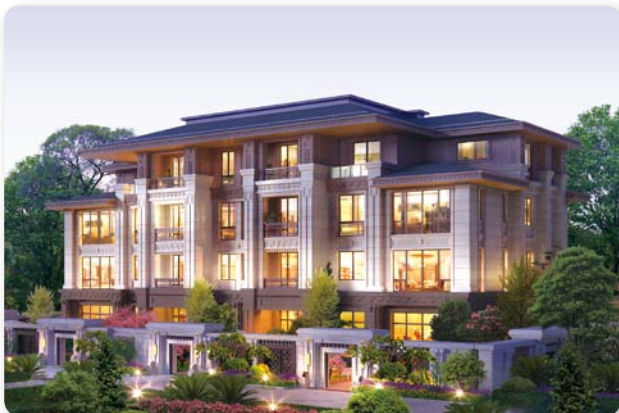
Zhengzhou Jiuru House
