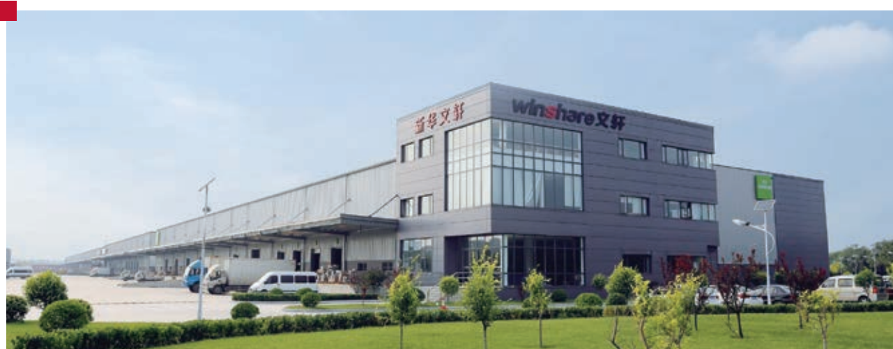
Our Northern China Logistics Centre completed construction and was put into use
