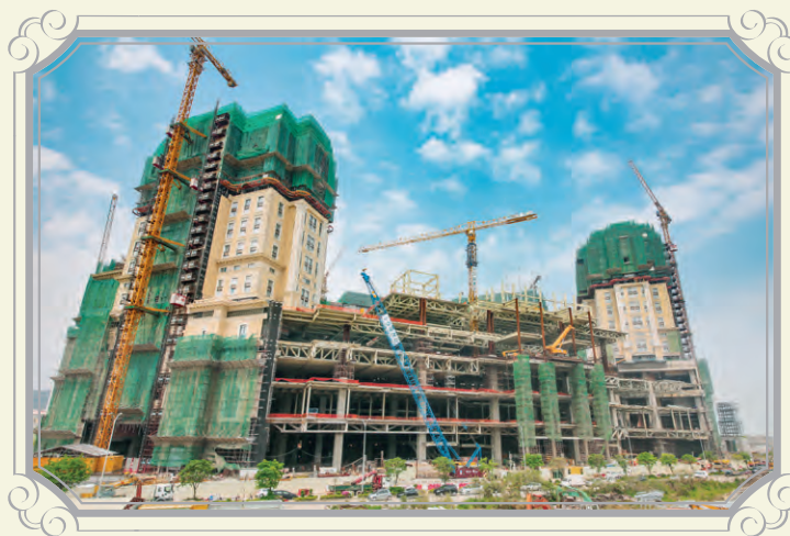
Construction in progress (photo taken in April 2017)
