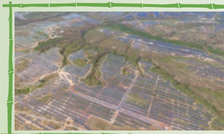
Aerial View of Datong National "Top Runner" Project
