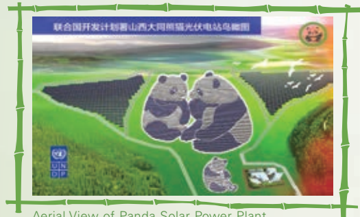
Aerial View of Panda Solar Power Plant
