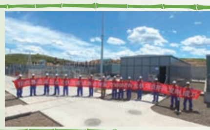
Datong National "Top Runner" Project Successfully Connected to Grid and Started Power Generation
