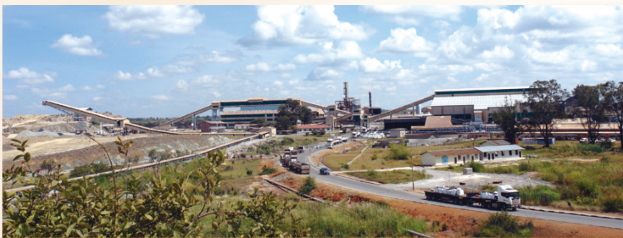
Panorama of Chambishi Copper Mine processing plant
