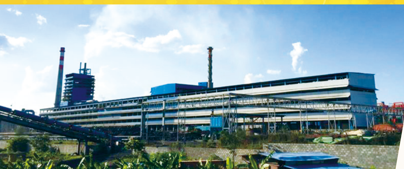
A general view of the exterior of Chambishi Copper Smelter
