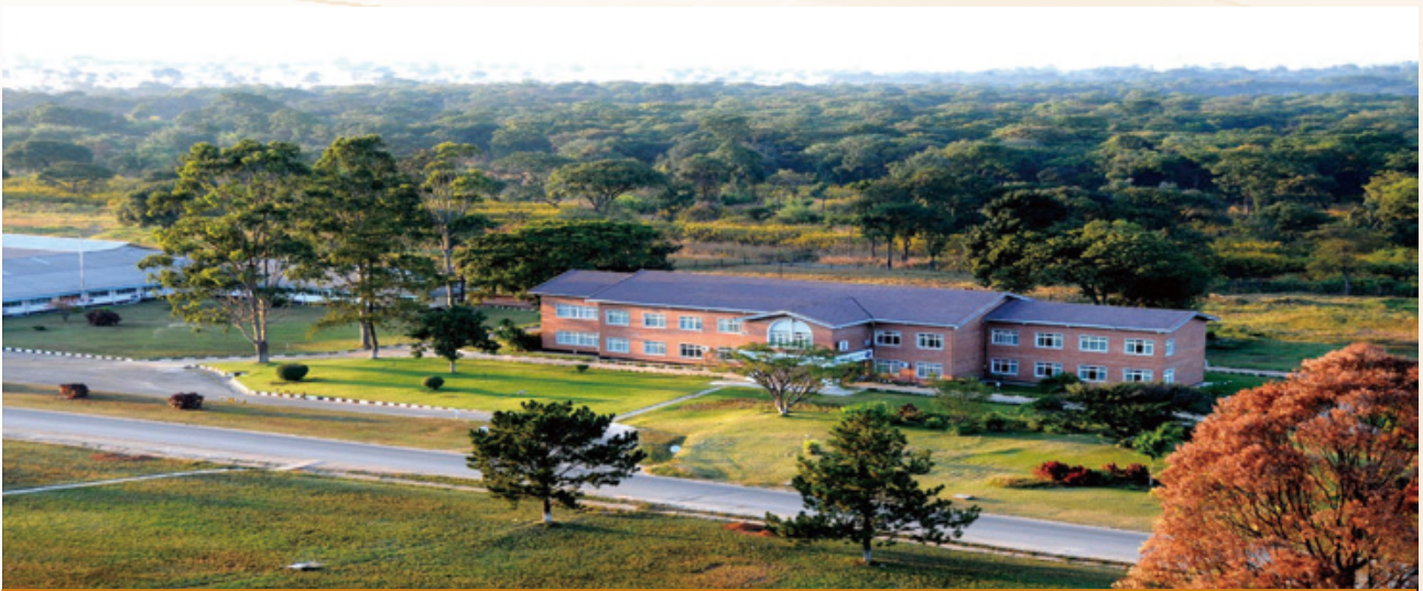
Central office building of NFCA in the green bush
