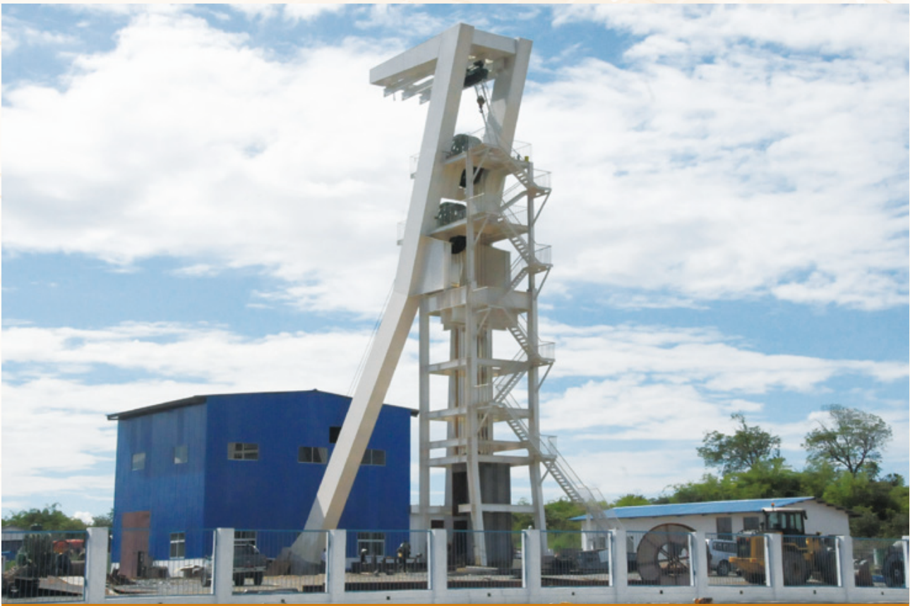
Central auxiliary shaft of Chambishi West Mine
