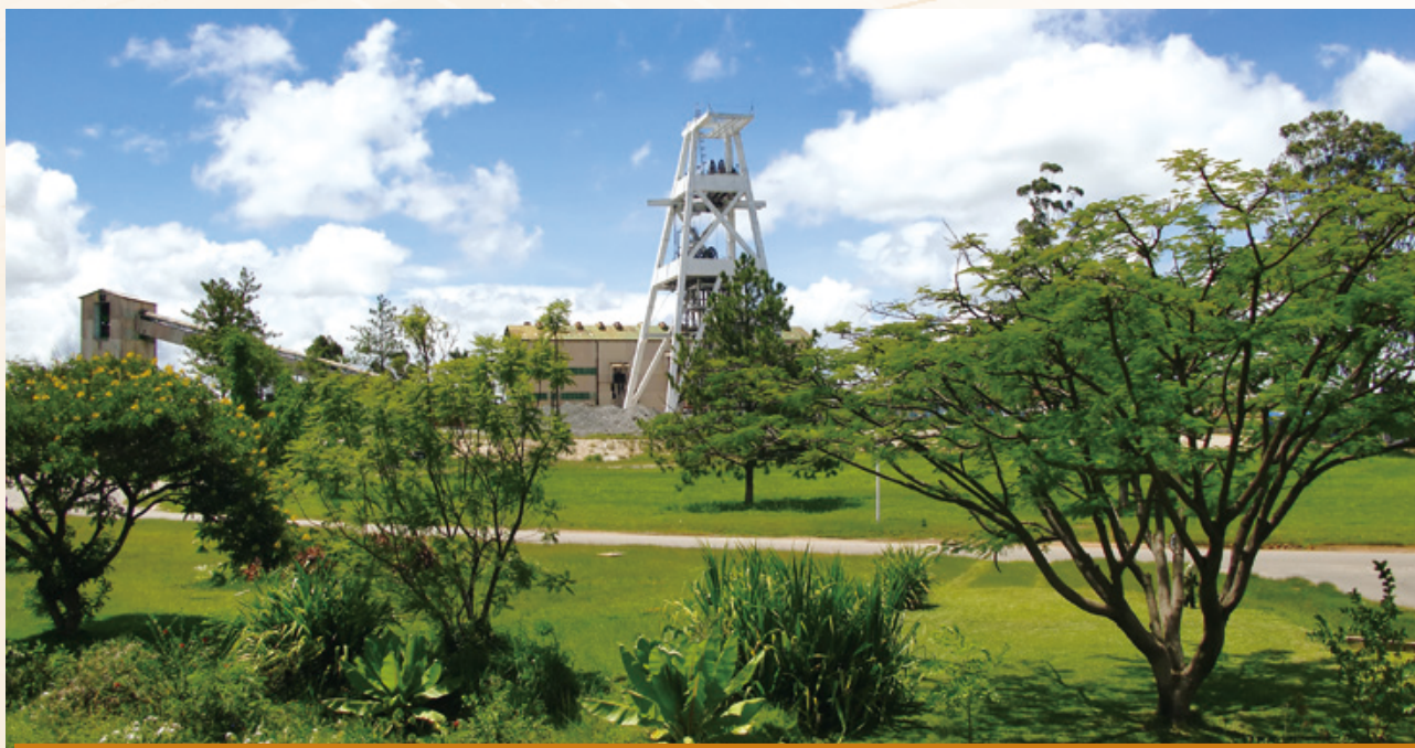
Main shaft of Chambishi Copper Mine
