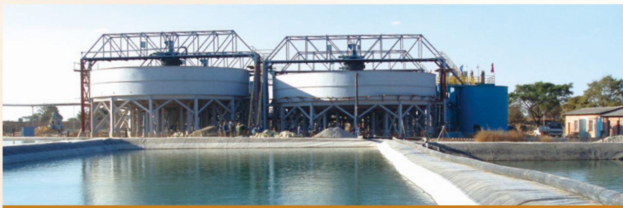
Settling pond for leaching
