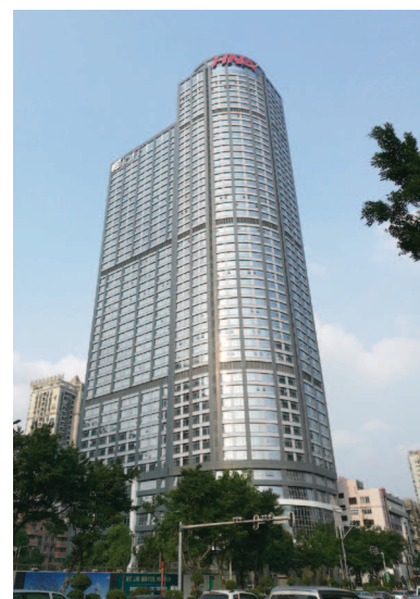
Tianhe Project – Outlook
