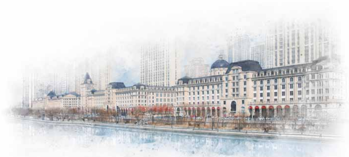
City Plaza (Tianjin)
