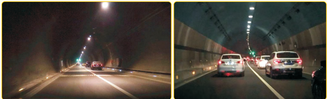
Chengyu Expressway Longquanshan Tunnel and Chengren Expressway Ereshan Tunnel after the energy saving reconstruction
