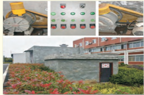
The wastewater centralized treatment facilities
