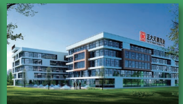
CT Tianqing's R&D Centre
