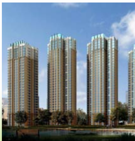
■ Residential towers of Regal Renaissance – superstructure works nearing completion (*)
