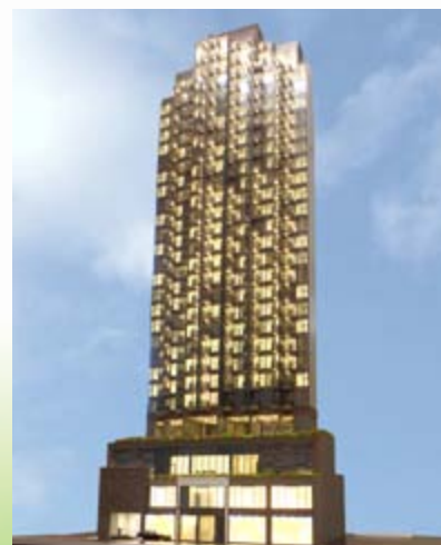
■ The Ascent, a commercial/residential development at No. 83 Shun Nin Road, Sham Shui Po, Kowloon, – superstructure works in progress (*)
