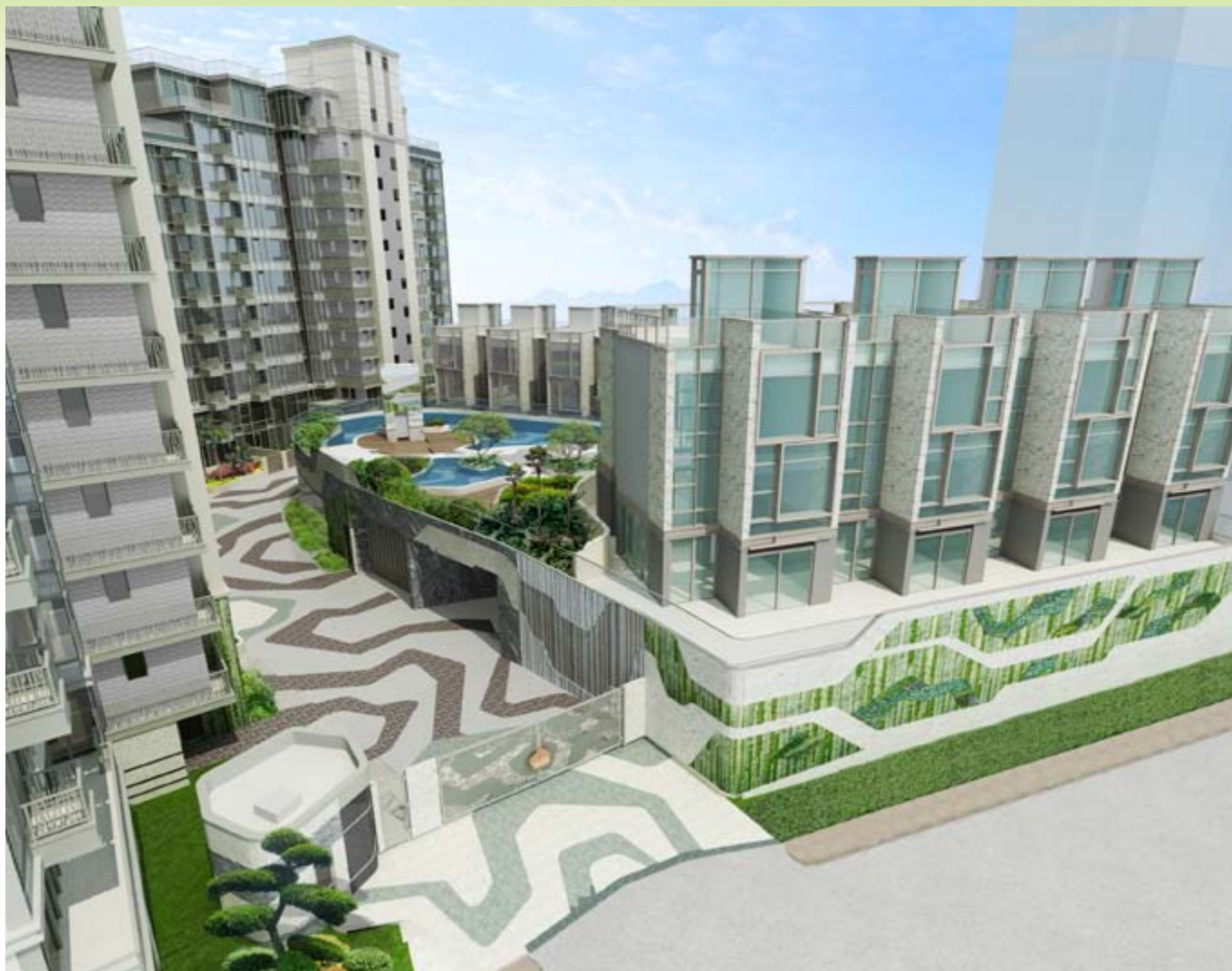
■ Luxurious residential development at Sha Tin Town Lot No. 578, Area 56A, Kau To, Sha Tin, New Territories – superstructure works in progress (*)
