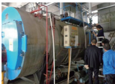
Figure 6. Installation of Non-invasive Electromagnetic Scale Control System 圖6. 安裝非嵌入式電磁波水垢清除系統
