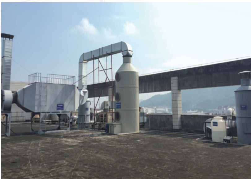
Figure 5. VOC's Treatment Facility 圖5. VOC處理廠
