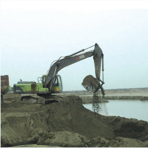
Comprehensive Utilization of Cement Mixture for Tailings 1 (Yangzhuang Iron Mine)
