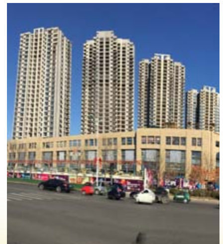
■ Residential and commercial portions of Regal Renaissance (*)
