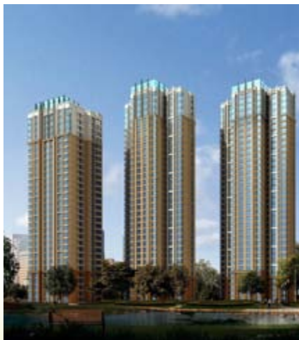
■ Residential towers of Regal Renaissance – superstructure works nearing completion (*)
