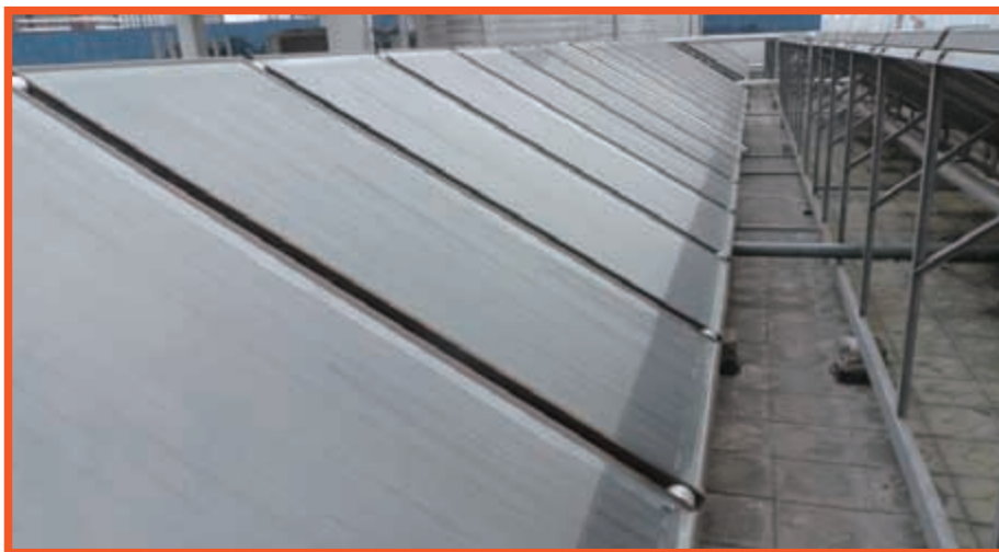
Figure 3: Solar Panels on the Rooftop of Our Staff Quarters
