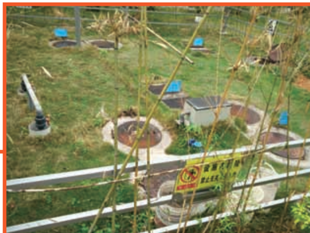
Figure 5: Sewage Purification Project within Factory Premises
