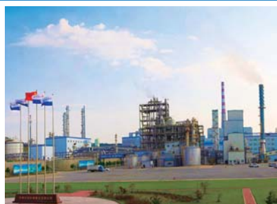
The production facilities in Heilongjiang
