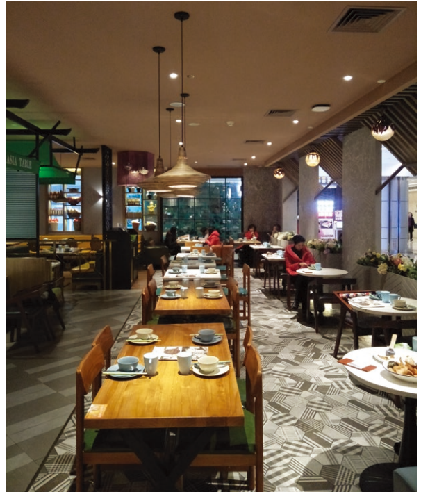
LED lighting project – Restaurant, PRC.
