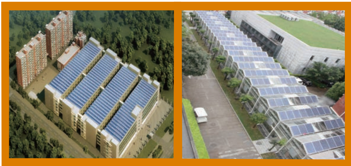
Solar Photovoltaic System on Rooftop of New Huizhou Factory
