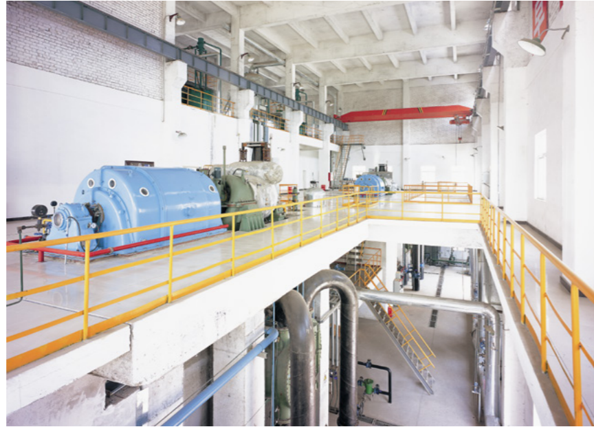
Low-heat residual heat power generation units
