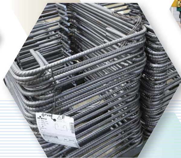
Bent Rebar with Traceability 彎曲鋼筋附追蹤機制
