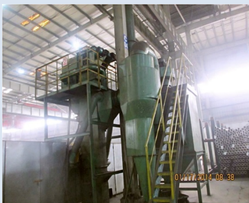
Sandblasting equipment before demolishing
