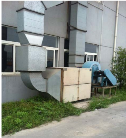
Environmental protection equipment for VOCs removal
