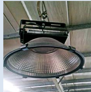
Lamp after retrofit
