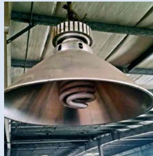
Lamp before retrofit
