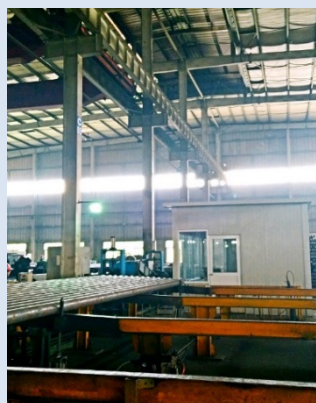
Sandblasting equipment after demolishing
