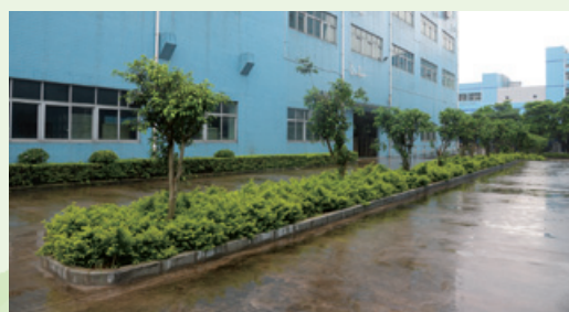
Location: Passageway between Block A2 and A3 位置：A2及A3座之間通道
