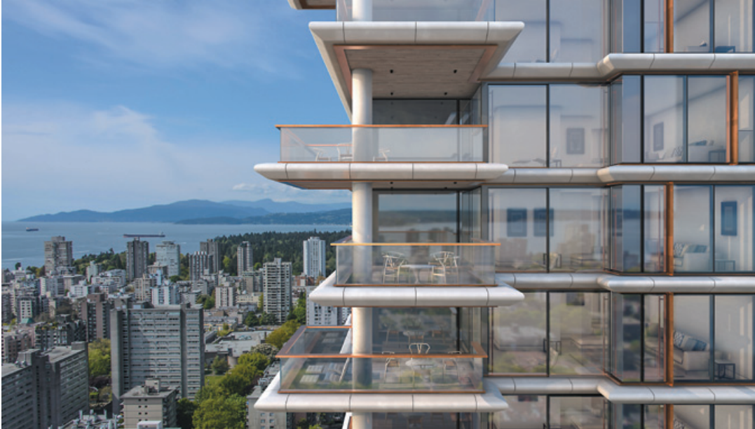
Residential re-development of Empire Landmark Hotel on Robson Street, Vancouver
