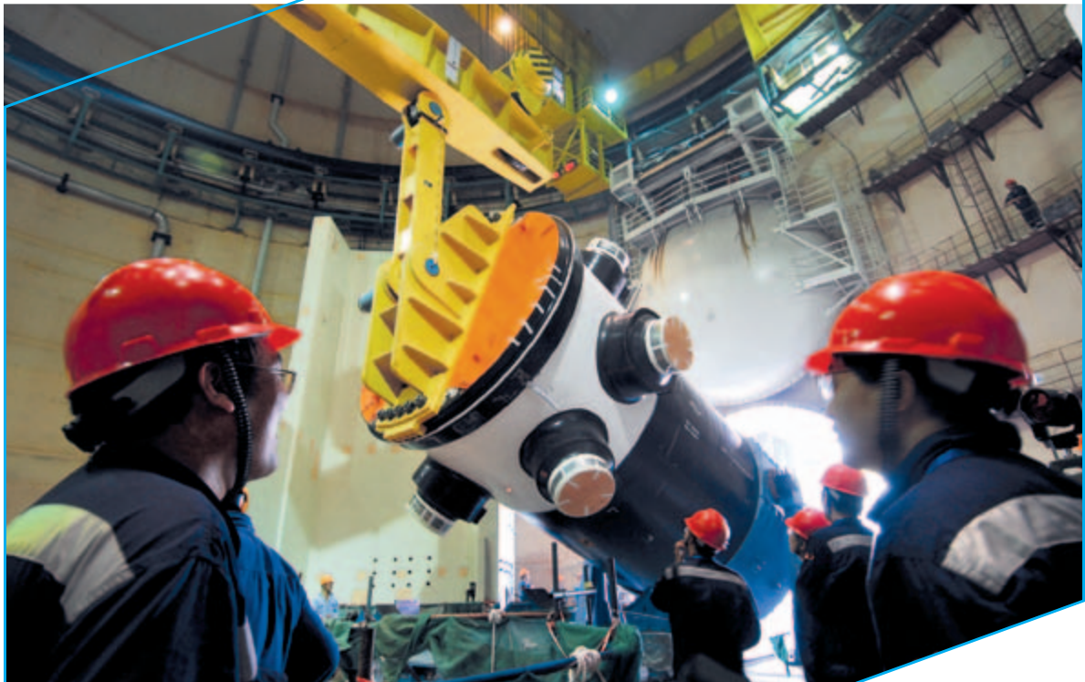
Equipment installation by engineering staff
