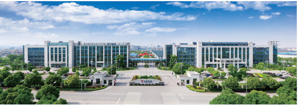
(The Group’s Lithium Battery Production Base)
