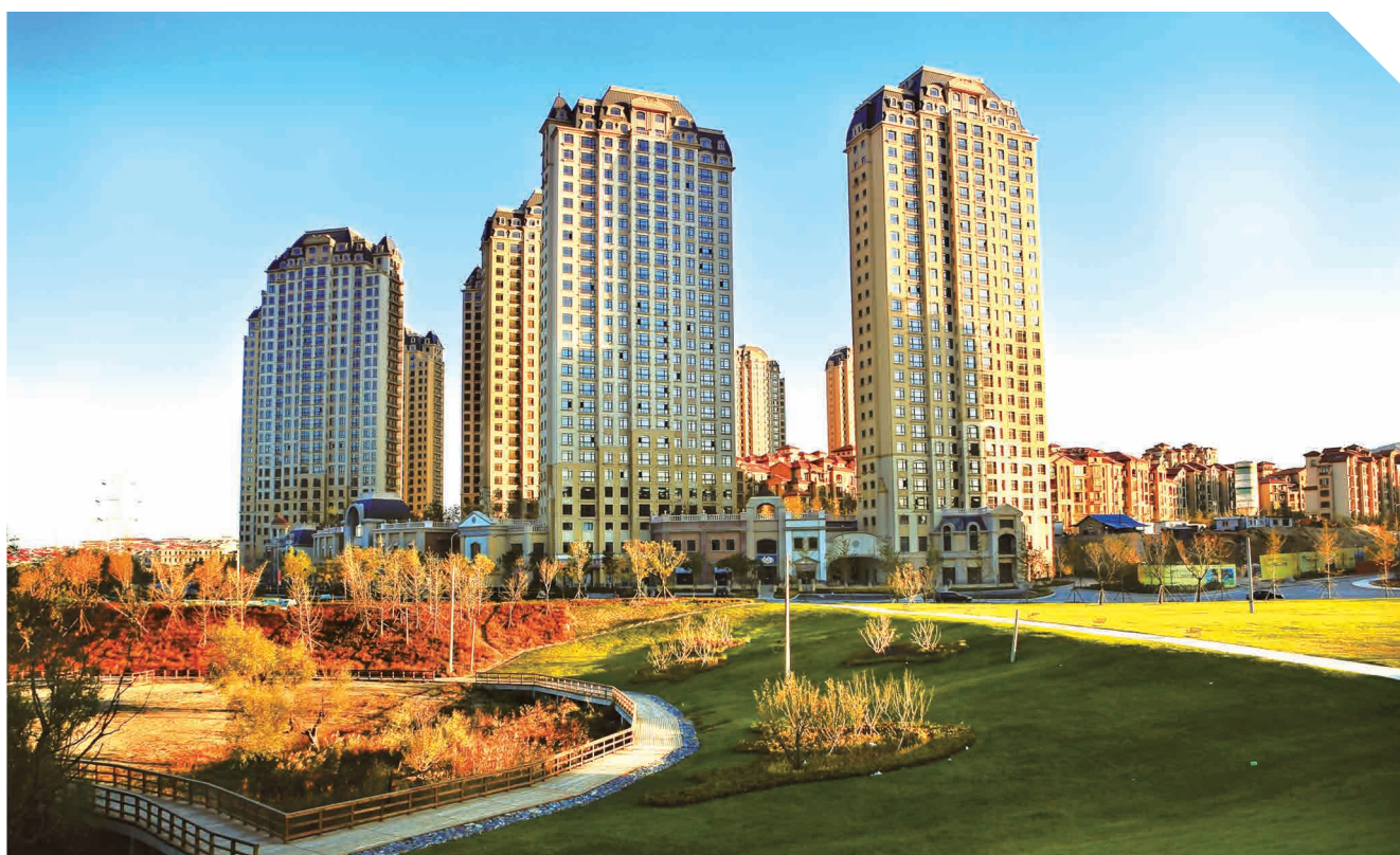
Residential project Qingwan in Dalian
