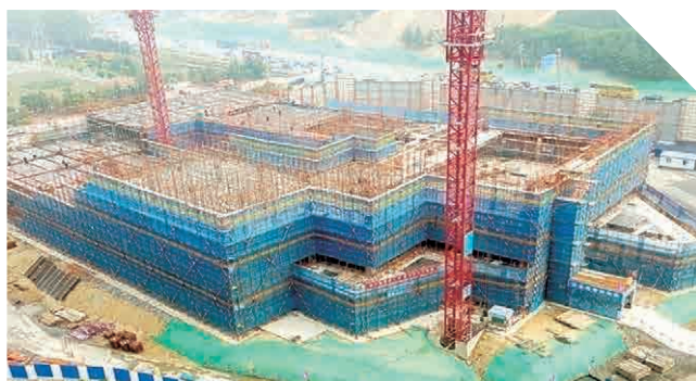
Construction of Eton International School
