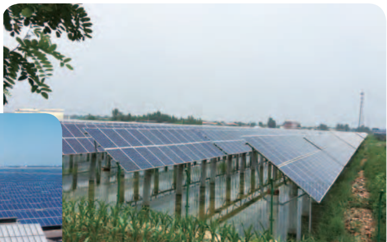
Laoling Tiejing Solar Power Project
