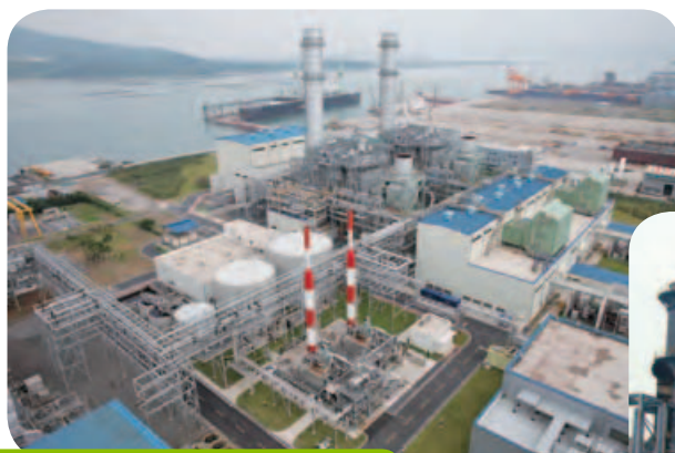
Yulchon Gas-fired Project (Phase II)
