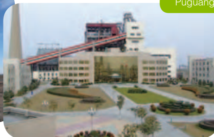
Puguang Coal-fired Project
