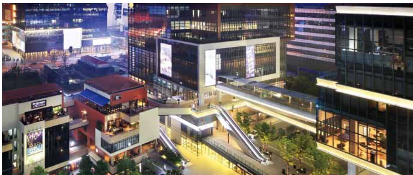
THE HUB has become the first stop for many passengers travelling through Hongqiao Transportation Hub
