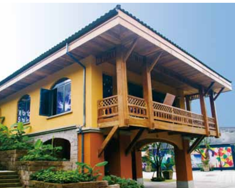
Chongqing Tiandi incorporates the traditional culture in its development
