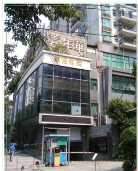
Facade of Xiyang Computer City 熹陽電腦城外景
