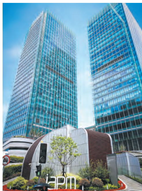
With their advantageous location atop IAPM and advanced facilities, the Shanghai ICC office towers appeal to multinationals from diverse sectors
