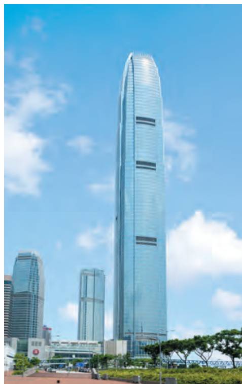
Superior specifications and full facilities place the IFC office towers among the most coveted business addresses in Hong Kong
