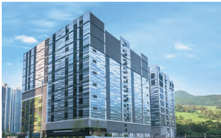
SUNeVision's MEGA Plus is the first purpose-built high-tier data centre in a designated zone of Hong Kong equipped with next-generation technology
