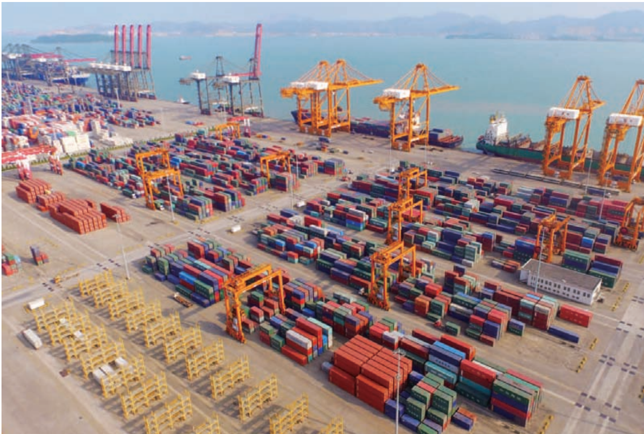
Xiamen Container Terminal
