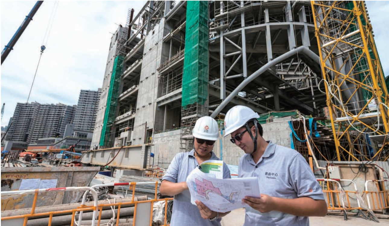
Together with our partners and suppliers, we build many of Hong Kong's iconic landmarks, including Xiqu Centre in West Kowloon.
