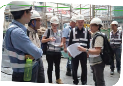
Regular management safety and health inspection
