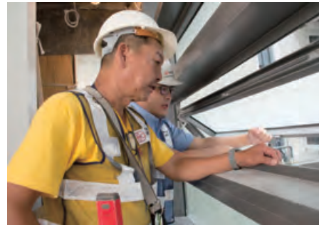
Quality check by site staff
