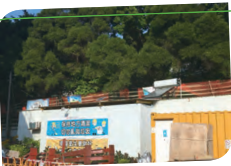
Renewable energy water heater system
