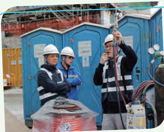
Safety aspects monitoring at site
