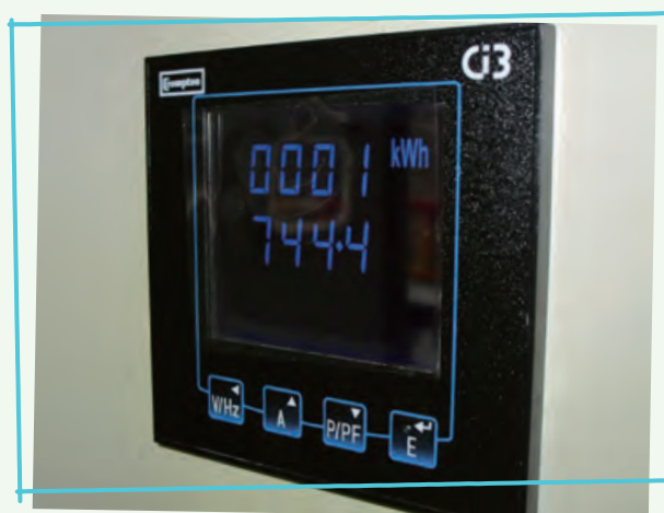
Energy monitoring system to help reduce the energy consumption
