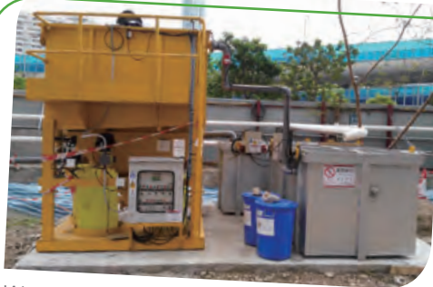
Wastewater treatment facility
