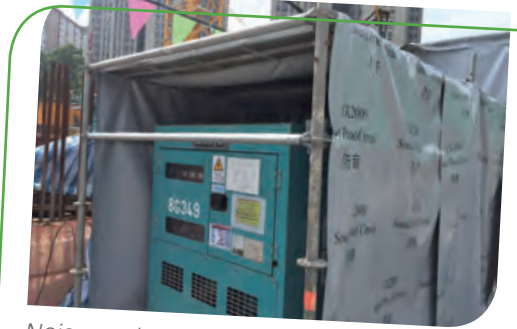
Noise enclosure for generator
