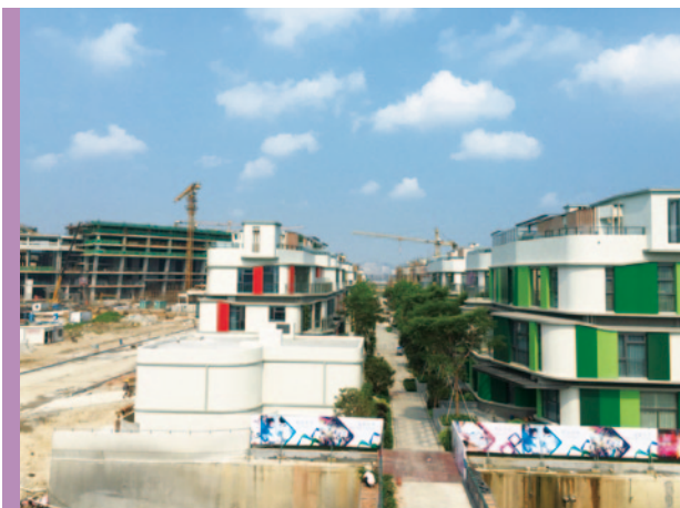
Hengqin Novotown Project Phase I
