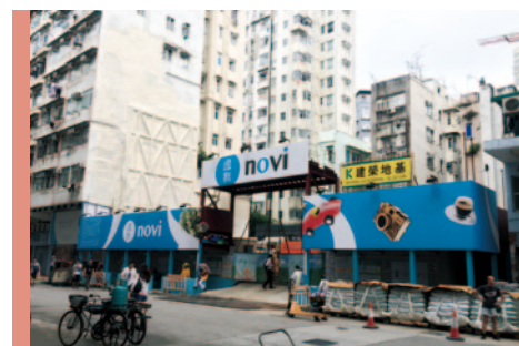
Latest construction progress of Novi
