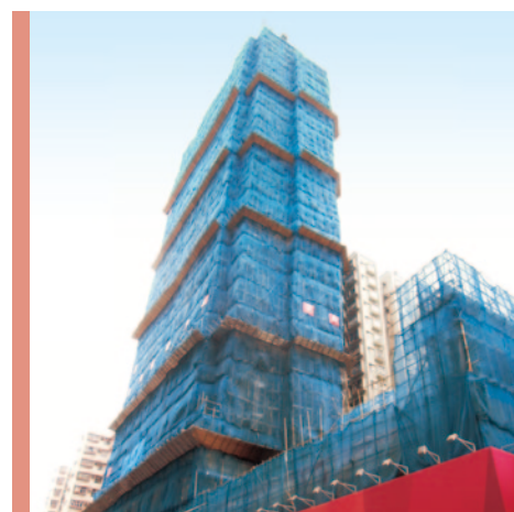
Latest construction progress of 93 Pau Chung Street
