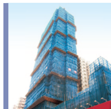
Latest construction progress of 93 Pau Chung Street
