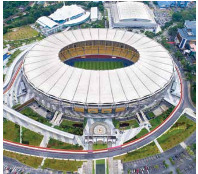
Refurbishment works of the Bukit Jalil National Sports Complex
