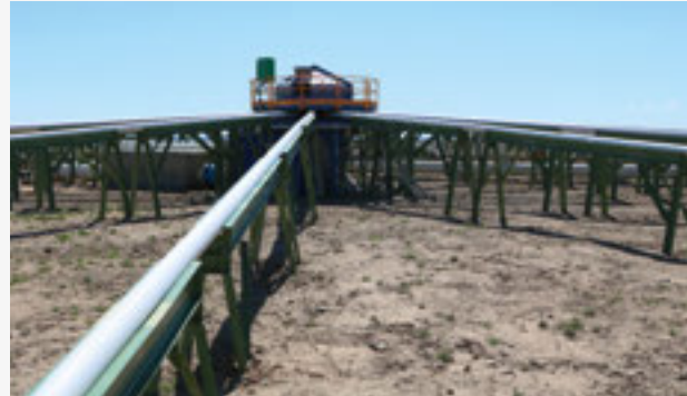
Aktogay tailings storage facility
