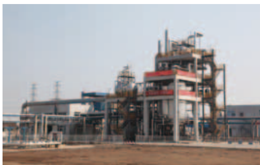
Changmao Lianyungang – Maleic anhydride production line with annual capacity of 10,000 tonnes using butane production method
