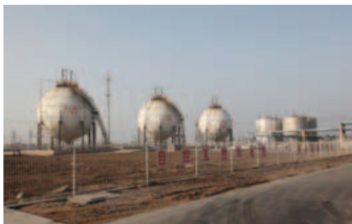
Changmao Lianyungang – Raw material (butane) storage tanks
