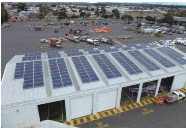
Solar panels installed on the roofs of Powercor's depots have cut carbon footprint and emissions.
