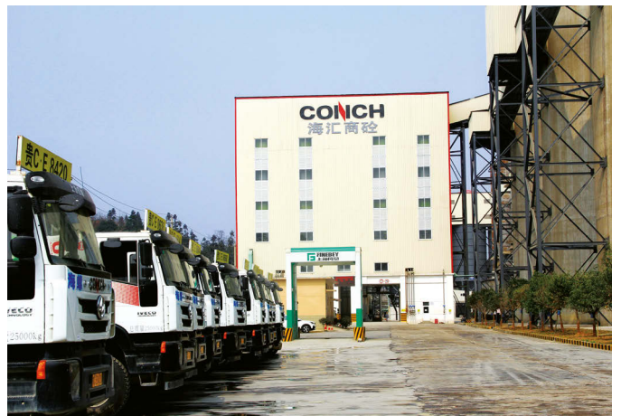
Commercial concrete project in Zunyi completed and put into operation
