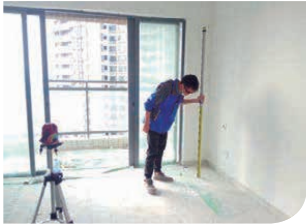
▲ Pre-occupation quality inspection
