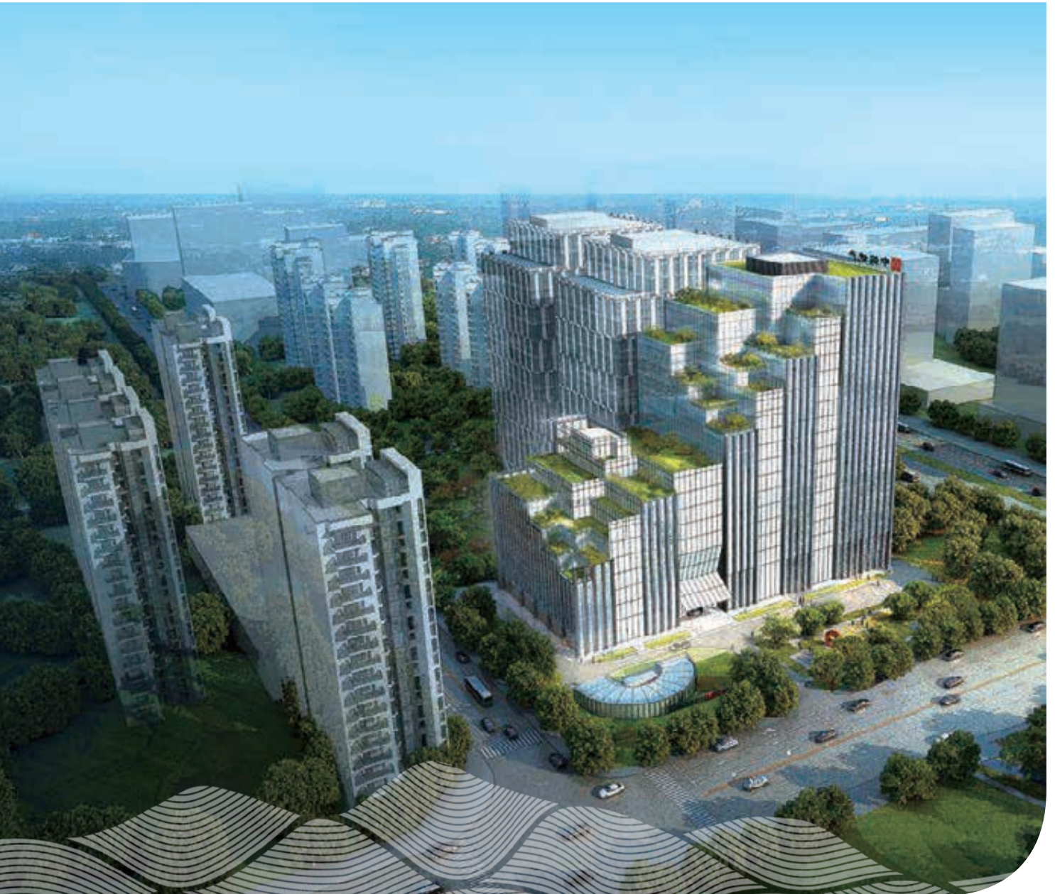
▲ Project JA at Shijingshan District, Beijing
