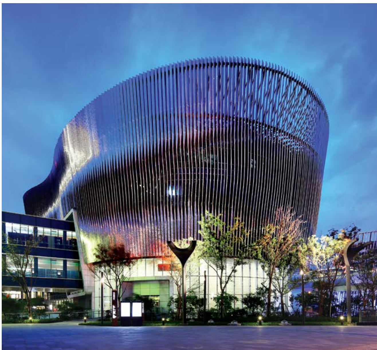
Night view of THE HUB
