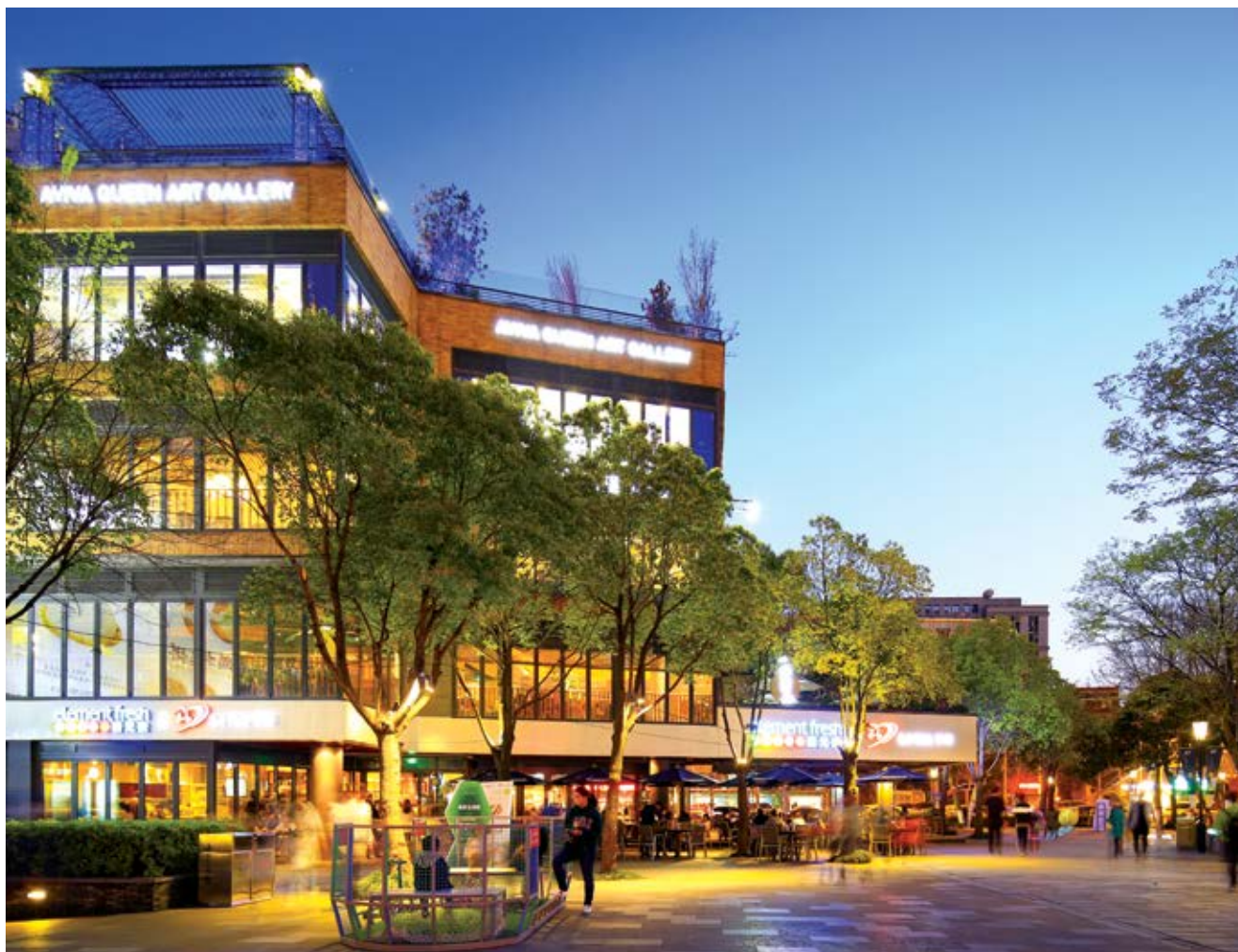
Wuhan Tiandi has matured with a mixture of commercial, office and residential elements
