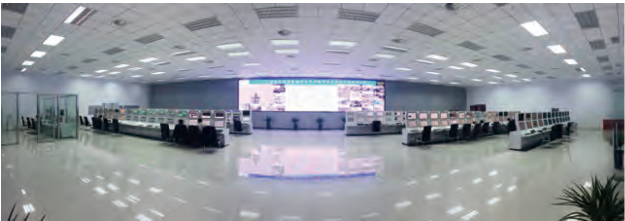
Interior of the Central Control Room
